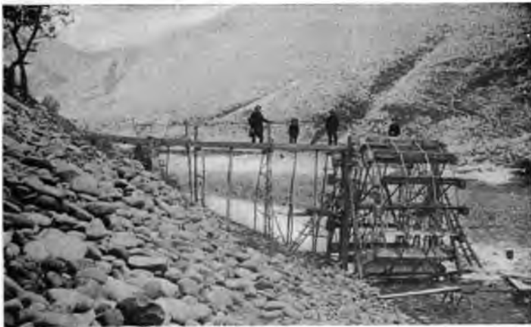
FIG. 20.—Current Wheel or Noria, Lifting Water from Salmon River for Irrigation.
